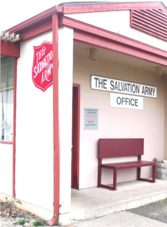
The current Salvation Army facility in Walla Walla, Wash. Photo by Donna Miranda
